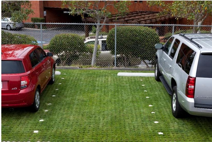
**Photo 1: Finished Drivable Grass® planted infill installation.**
