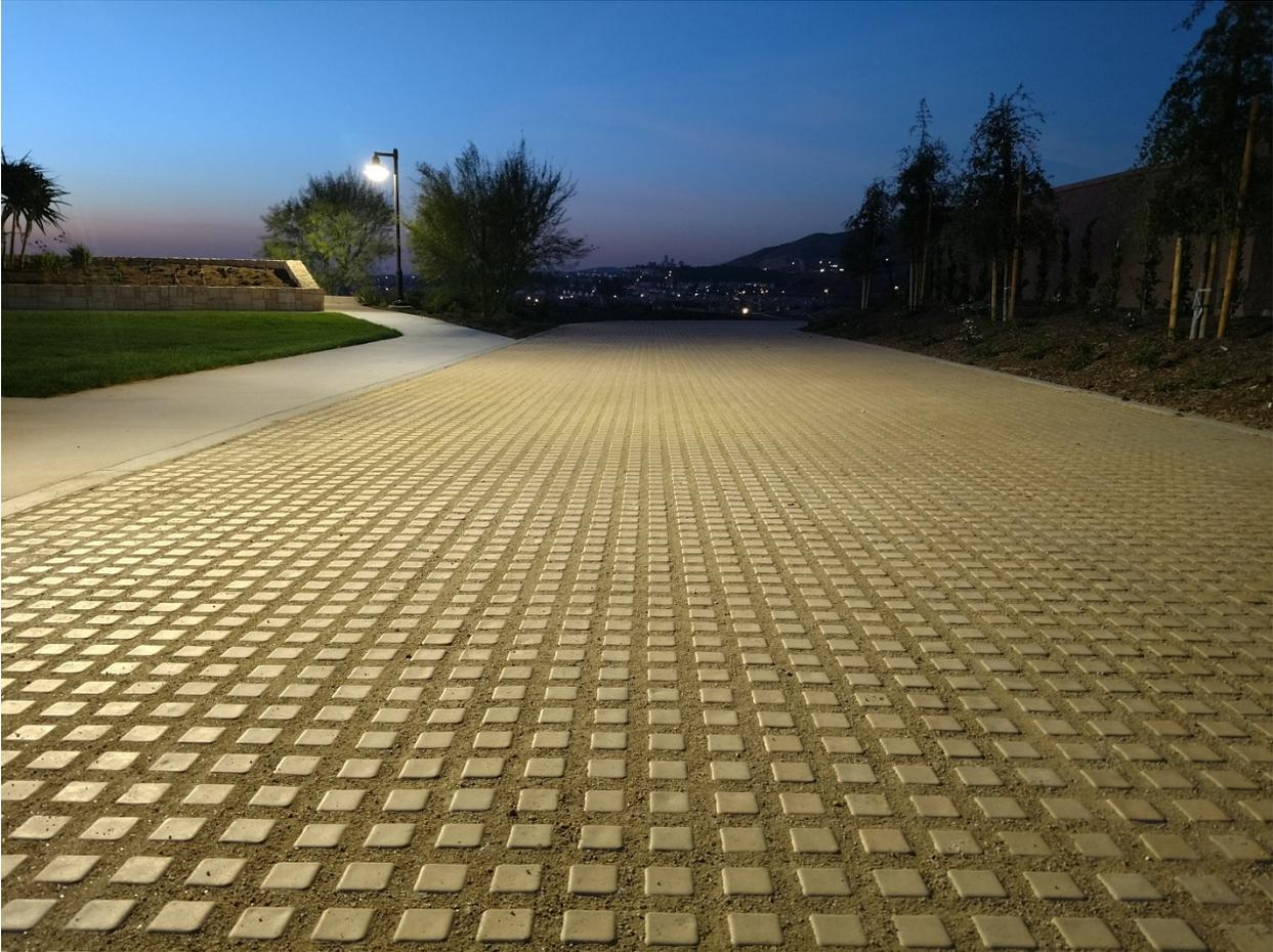
**Photo 5: Finished Drivable Grass® dry infill installation.**
