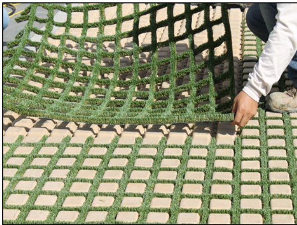
Photo 5: Pre-Fit Installation of Drivable Turf.
