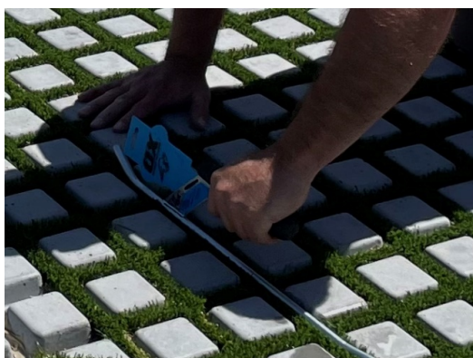
Photo 10: sled brick jointer used to adhere turf
