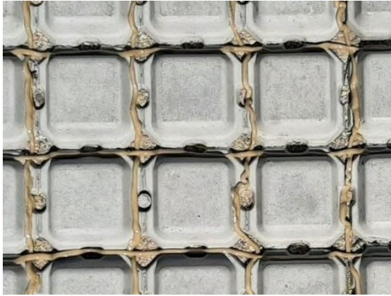
Photo 8: Option 2 Adhesive Application
