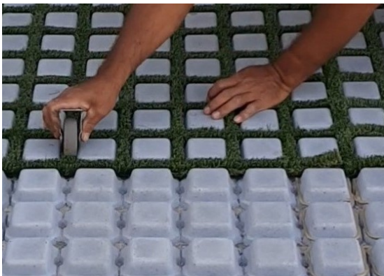
Photo 9: Wheel used to adhere turf
