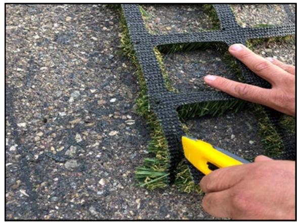
Photo 6: Backing cut for an edge termination
