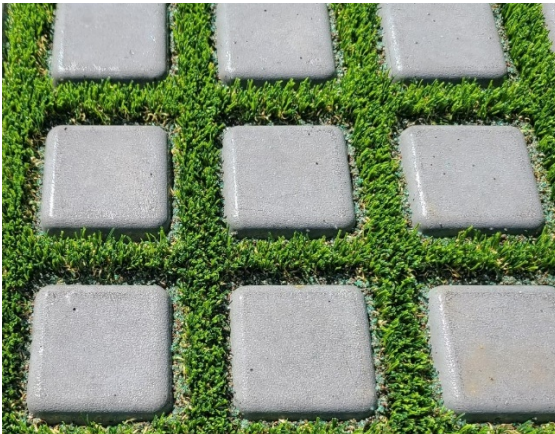
Photo 11: Finished installation using colored sand
