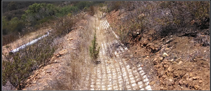
Typical Drainage Swale Detail
