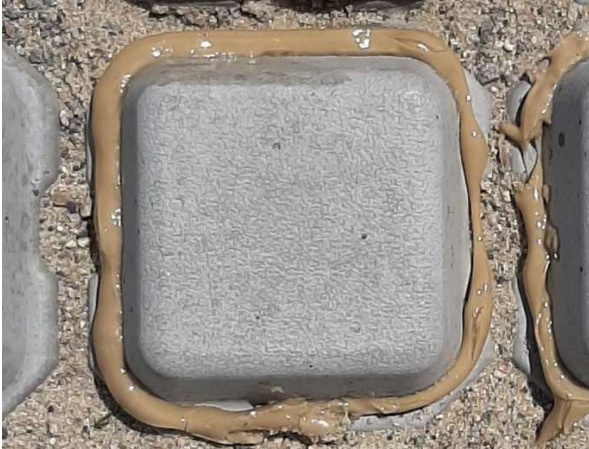
Photo 7: Option 1 Adhesive Application
