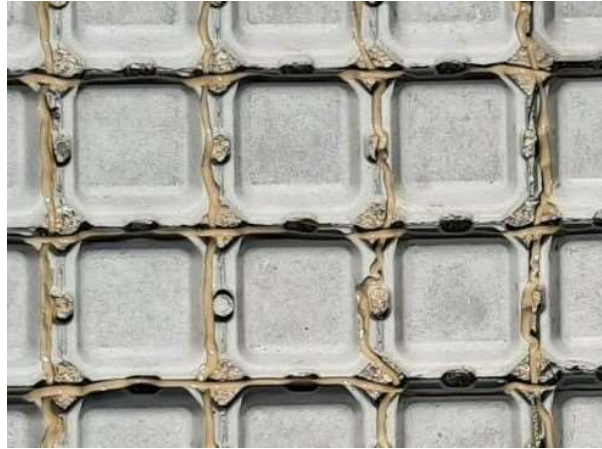
Photo 8: Option 2 Adhesive Application
