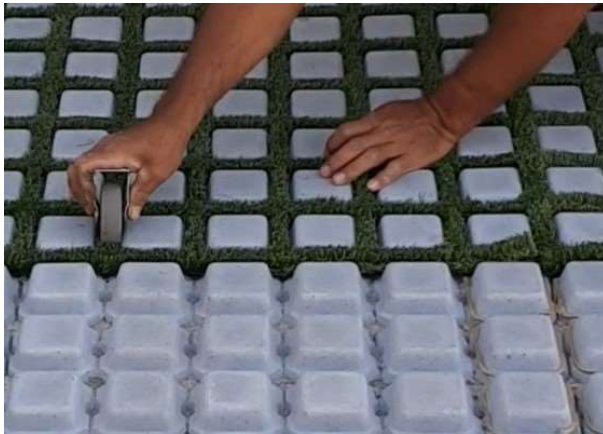
Photo 9: Wheel used to adhere turf
