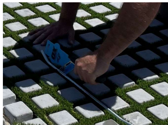
Photo 10: sled brick jointer used to adhere turf
