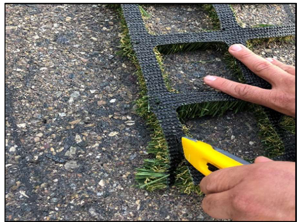
Photo 6: Backing cut for an edge termination
