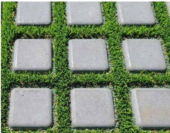
Photo 11: Finished installation using CamoFill®
