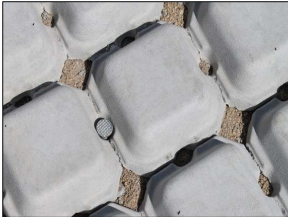
Photo 3: Spike driven into base of mat.
