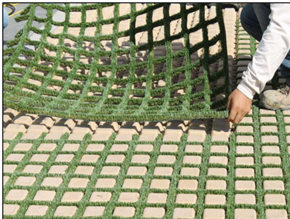
Photo 5: Pre-Fit Installation of Drivable Turf.
