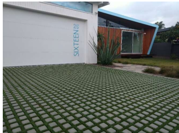
Photo 12: Finished Drivable Turf® installation
