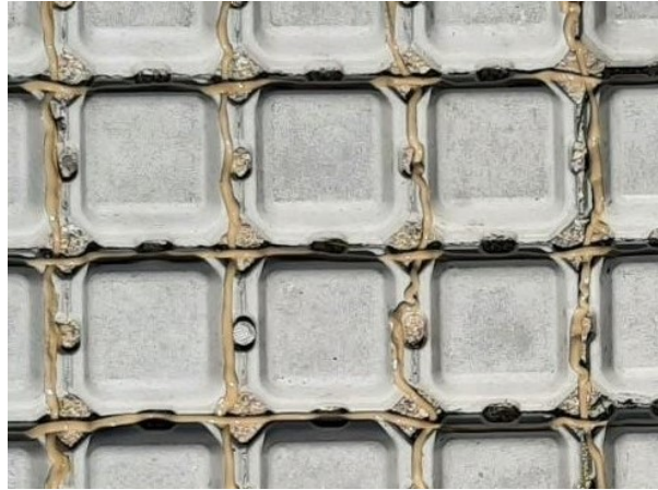
Photo 8: Option 2 Adhesive Application
