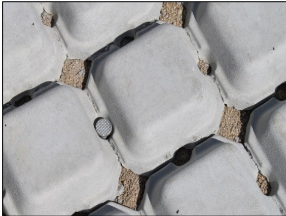
Photo 3: Spike driven into base of mat.
