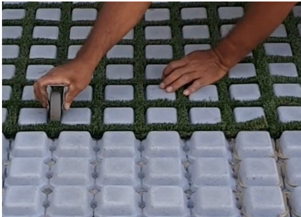
Photo 9: Wheel used to adhere turf
