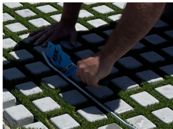
Photo 10: sled brick jointer used to adhere turf
