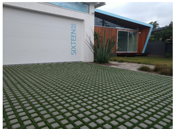
Photo 12: Finished Drivable Turf® installation
