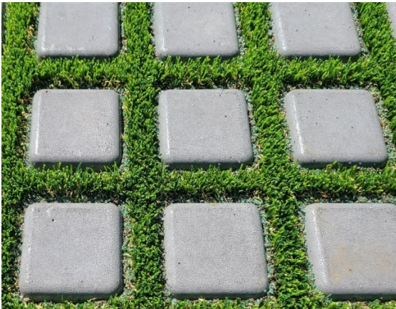
Photo 11: Finished installation using colored sand
