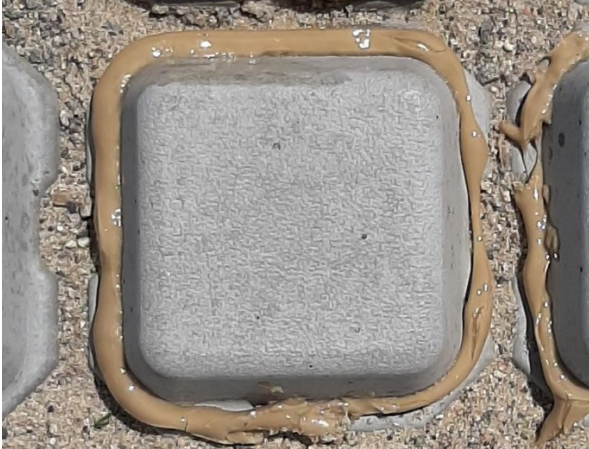
Photo 7: Option 1 Adhesive Application
