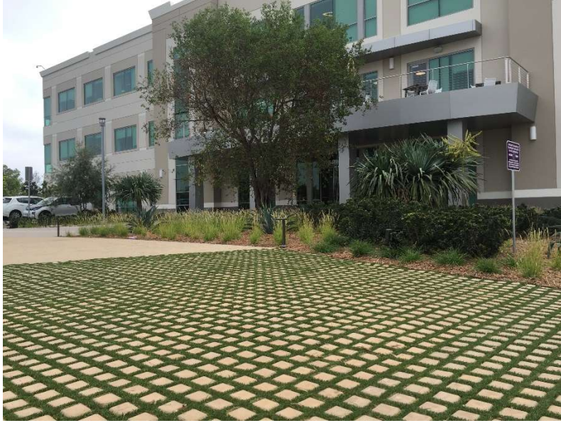
Photo 11: Finished Drivable Turf® installation.
