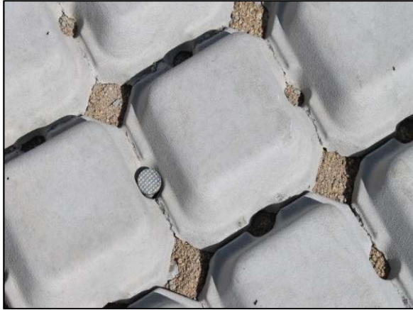
Photo 3: Spike driven into base of mat.
