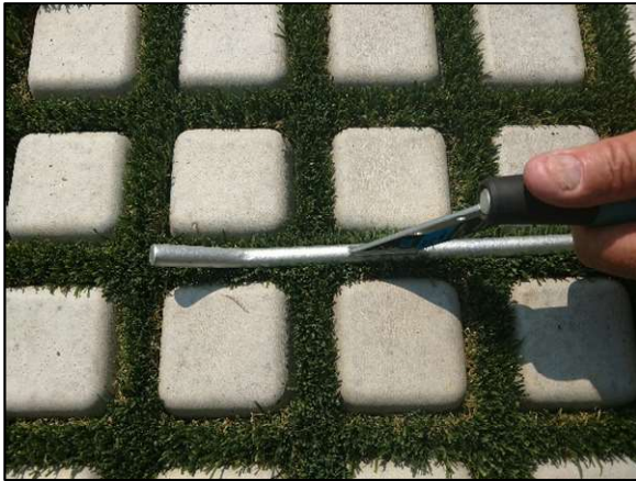
Photo 9: Pressing Drivable Turf® firmly into position with a heavy sled brick jointer
