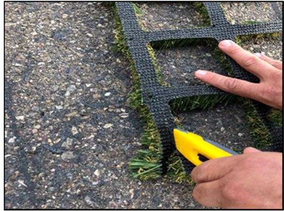
Photo 6: Backing cut for an edge termination
