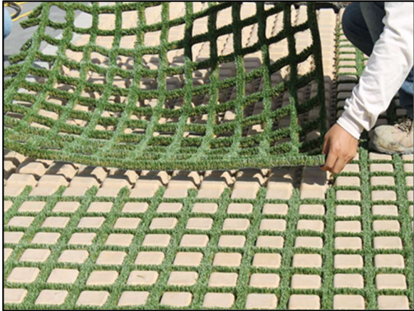
Photo 5: Pre-Fit Installation of Drivable Turf.
