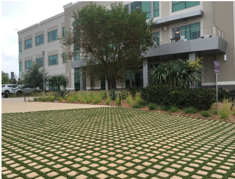
Photo 11: Finished Drivable Turf® installation.
