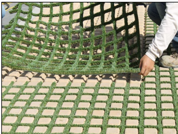
Photo 5: Pre-Fit Installation of Drivable Turf.
