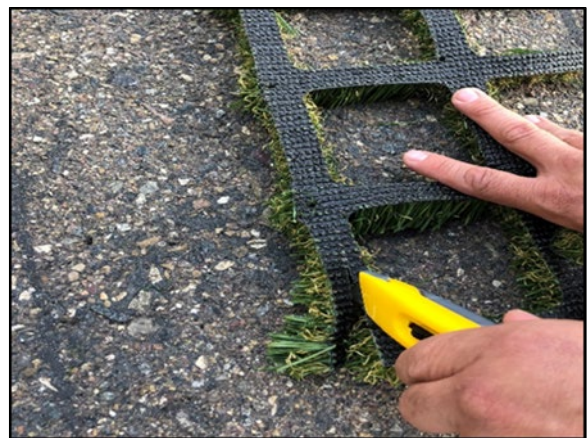
Photo 6: Backing cut for an edge termination
