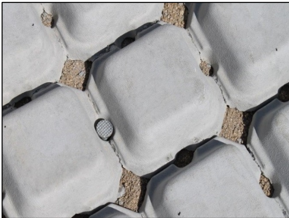
Photo 3: Spike driven into base of mat.
