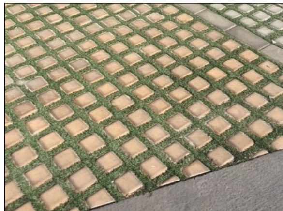
Photo 10: Sand broomed into Drivable Turf ®
