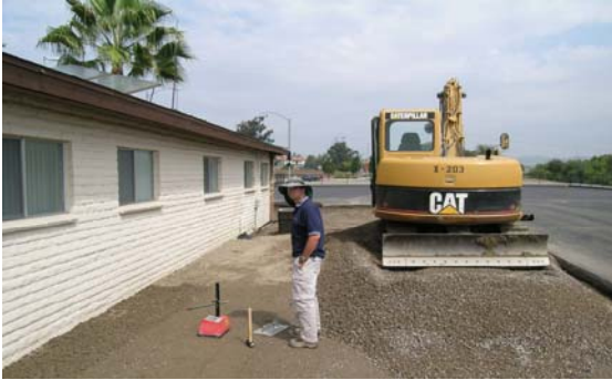
Figure-8: Density Testing of Aggregate Base
