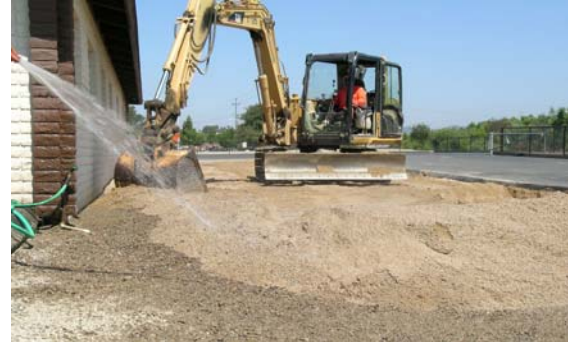
Figure-9: Placement of sand/organic layer
