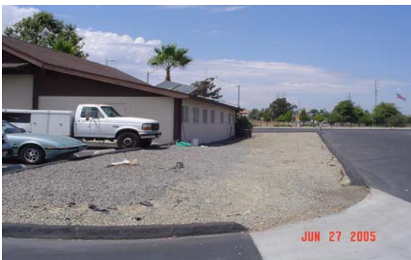
Figure-5: Fire Truck Wash Area – Before
