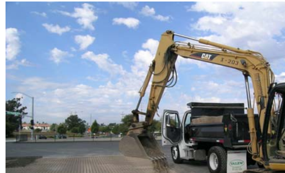
Figure-11: Infill Placement
