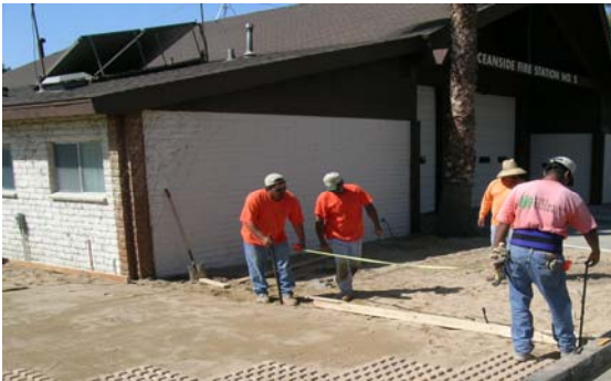
Figure-10: Mat Installation
