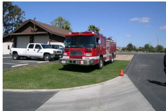
Figure-6: Fire Truck Wash Area - After
