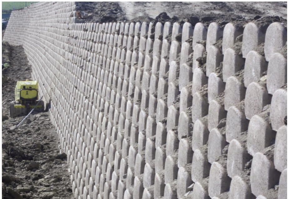
Verdura Wall supporting the Target Store site.
