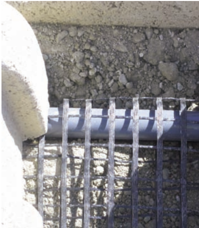
Verdura Wall positive connection
