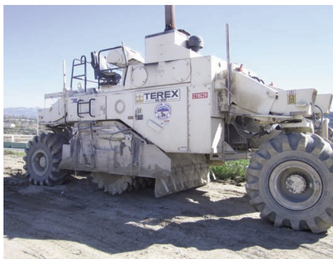
Lime treatment soil mixer.
