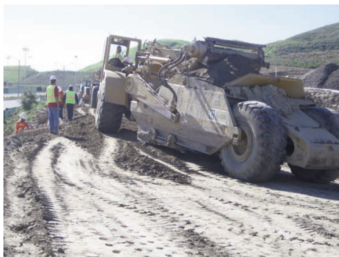
Scraper bringing lime treated soil to MSE Wall.
