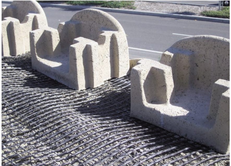
Miragrid® 8XT in lime treated soil.
