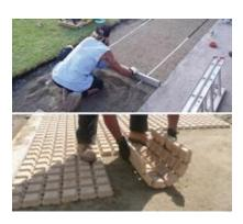
The grid inside the Drivable Grass® mats can be cut with a utility knife or chisel to fit site conditions. At terminating edges or curved installations, the mats should be fit with a masonry blade on a rotary saw.
