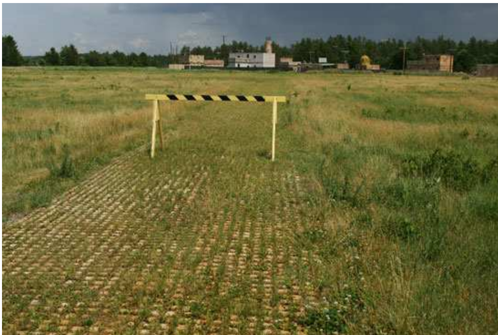
Driveable grass, pictured near the Urban Complex Training Site on North Post, provides improved access to vehicles and equipment, while helping to reduce environmental damage. (Photo by Rob Schuette)
