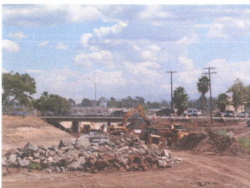
Fig. 5 – Concrete/ Earthen Interface
