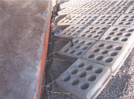
Fig. 24 - Eyebolt and Cable Tie-In
