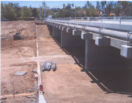
Fig. 11 – Olive Lane Bridge
