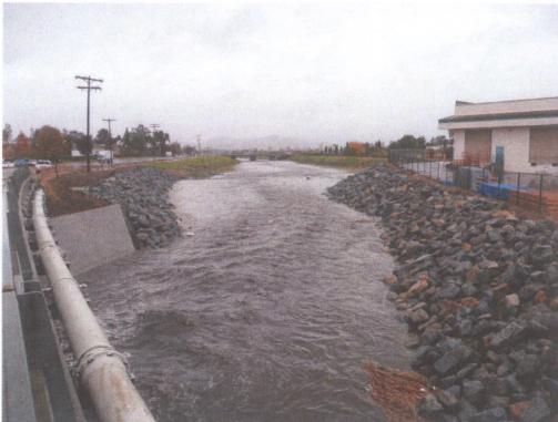
Fig. 29 – Energy Dissipater during Storm Event
