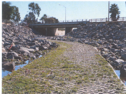
Figs. 31 and 32 – Energy Dissipater after Runoff Event - Enviroflex ® as part of Sustainable Channel Design
