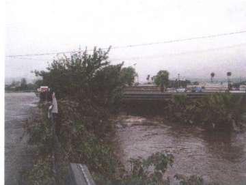
Fig. 3 – Mission Gorge Road Bridge
