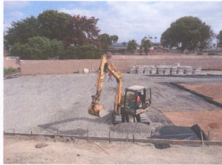
Fig. 18 – Fabric and Gravel Placement
