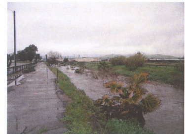
Fig. 4 – Near Overtopping of Banks
