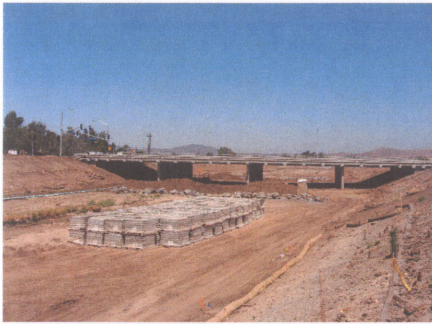
Fig. 17 – Product Delivered and Stored
