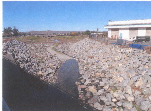
Fig. 30 – Energy Dissipater after Runoff Event
