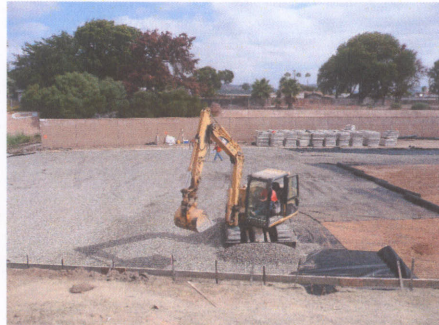
Fig. 18 – Fabric and Gravel Placement
