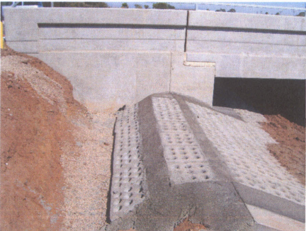
Fig. 26 – Top of Slope Anchor
