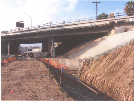
Fig. 8 – Concrete/ Earthen Interface
