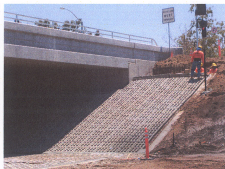
Fig. 13 – 2:1 Slope at Olive Lane
