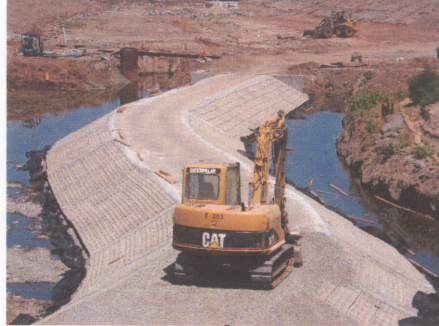
Fig. 9 – Enviroflex ® Access Road
