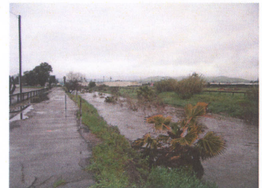
Fig. 4 – Near Overtopping of Banks
