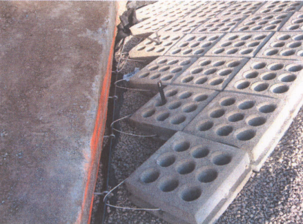
Fig. 24 - Eyebolt and Cable Tie-In
