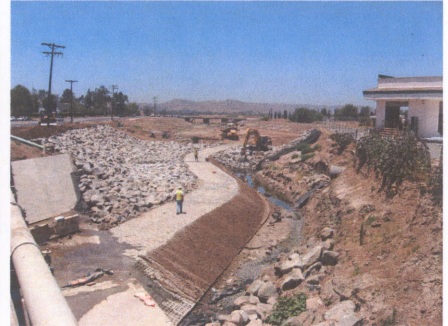
Fig. 10 – Rip Rap Placement
