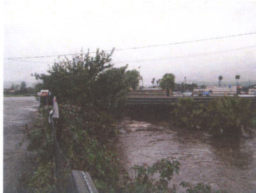
Fig. 3 – Mission Gorge Road Bridge
