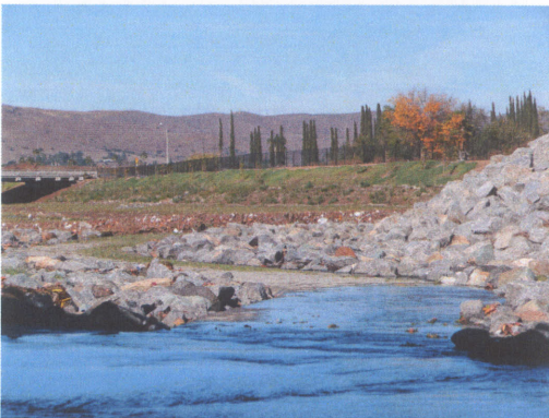
Figs. 31 and 32 – Energy Dissipater after Runoff Event - Enviroflex ® as part of Sustainable Channel Design
