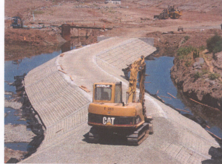
Fig. 9 – Enviroflex ® Access Road
