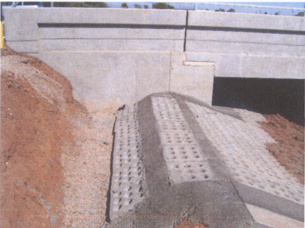
Fig. 26 – Top of Slope Anchor
