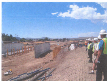
Fig. 6 – New Olive Lane Bridge
