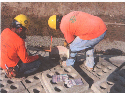
Fig. 23 – Saw-Cut Corners and Joints
