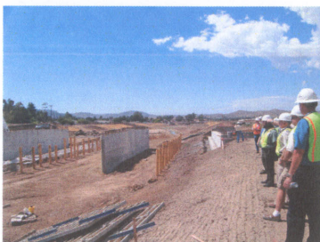
Fig. 6 – New Olive Lane Bridge
