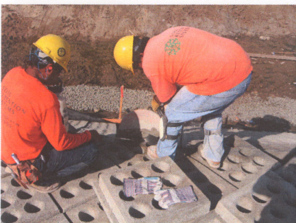
Fig. 23 – Saw-Cut Corners and Joints
