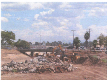
Fig. 5 – Concrete/ Earthen Interface
