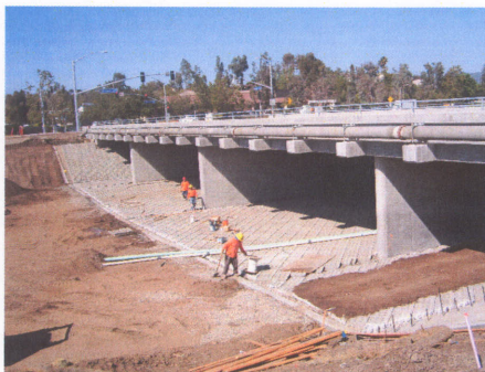
Fig. 12 – Enviroflex ® Installed under Olive Lane
