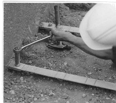
Figure 12. Fill spreading and reinforcement connection.
