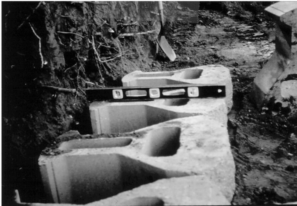
Figure 80. Checking facing element batter and alignment.
