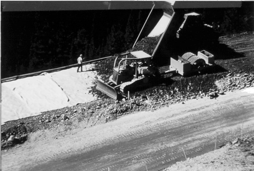
Figure 83. Placement of reinforced backfill.
