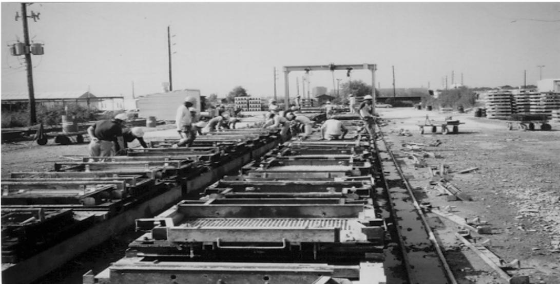
Figure 77. Casting yard for precast facing elements.
