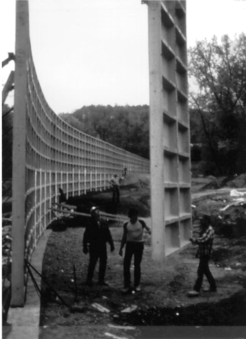
Figure 81. Full height facing panels require special alignment care.
