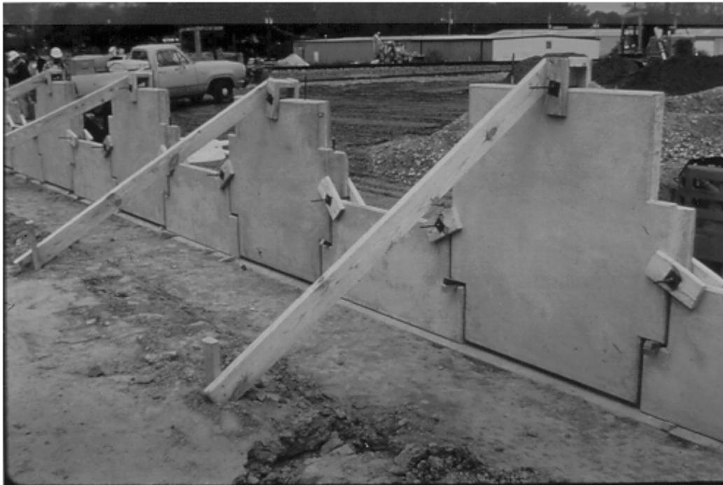
Figure 82. Setting first row of precast facing elements.
