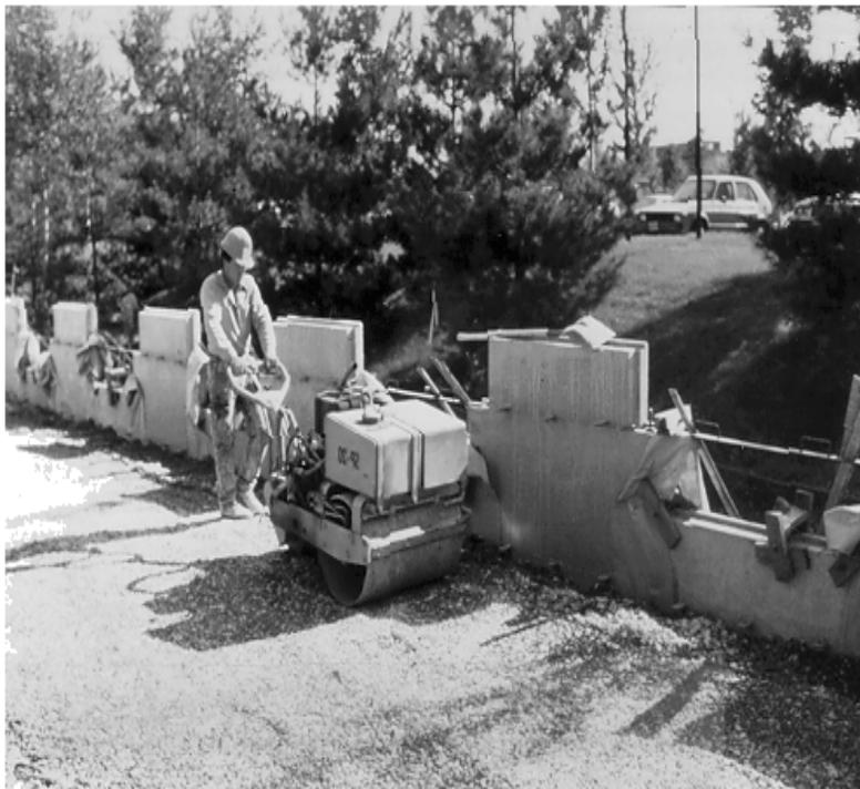
Figure 84. Compaction equipment showing: a) large equipment permitted away from face; and b) lightweight equipment within 1 m of the face.
