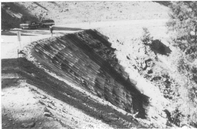
Figure 17. Reinforced slope construction; a) geogrid and fill replacement; b) soil fill erosion control mat placement; and c) finished, vegetated 1:1 slope.
