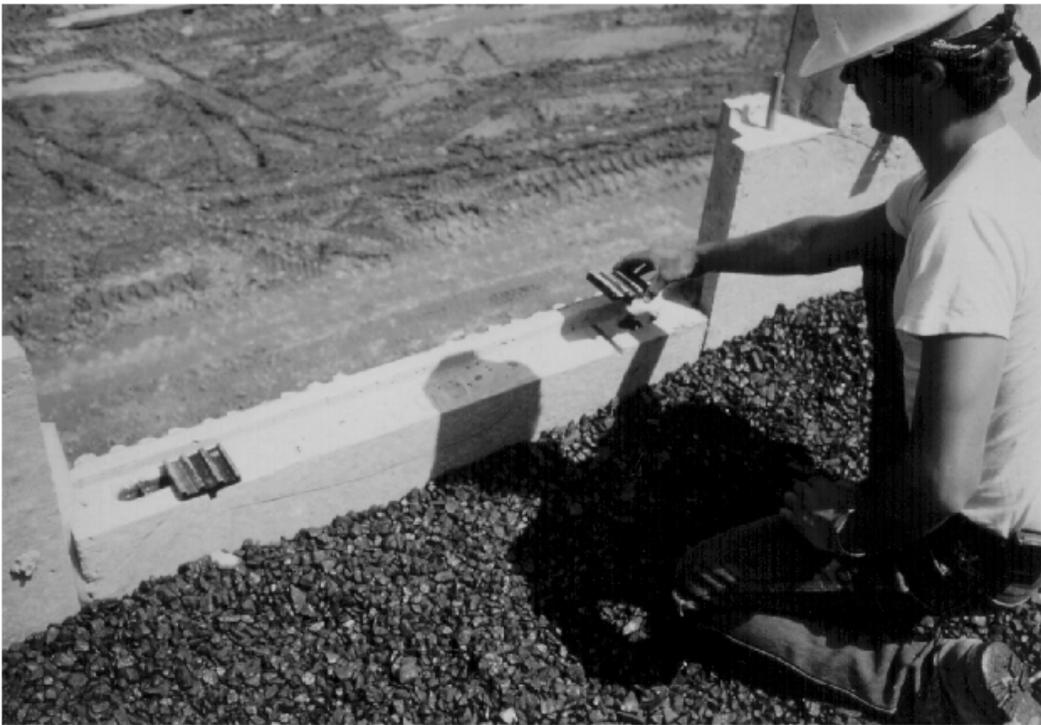
Figure 86. Geotextile joint cover and neoprene pads.
