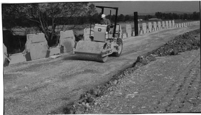
Figure 13. Compaction of backfill.
