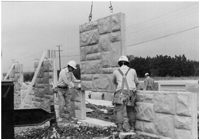
Figure 11. Erection of precast panels.
