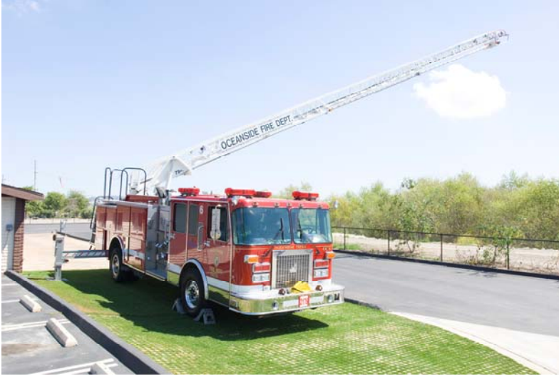
Finished test area was done with three different infills: cement stabilized gravel, sod, and a seeded portion.
