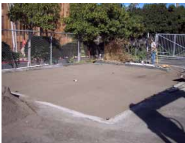
Fig. 5 – Tamped Sand Bedding
