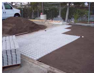
Fig. 6 – Drivable Grass ® Installation
