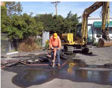
Fig. 2 – Removal of Asphalt
