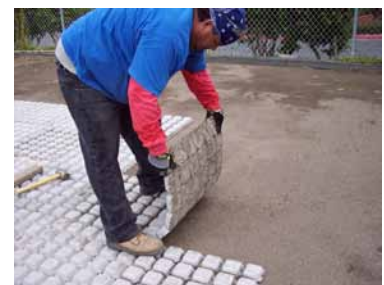
Fig. 7 – Drivable Grass ® Installation
