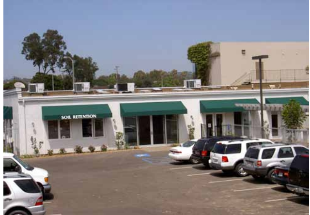
Fig. 1 – Soil Retention Headquarters Parking Lot
