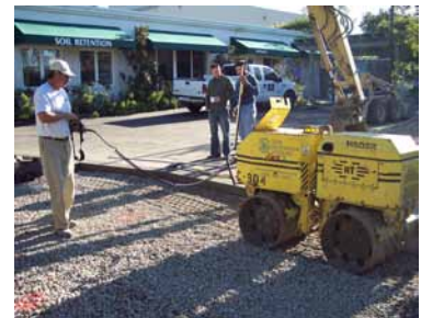
Fig. 4 – Compaction of Subgrade
