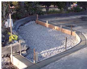
Fig. 3 – Crushed Gravel Subgrade
