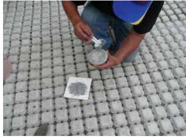
Fig. 9 – Installation of Bott's Dots
