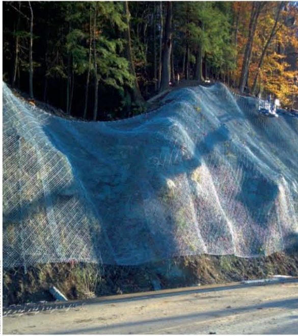
AMERITECH SLOPE CONSTRUCTORS
