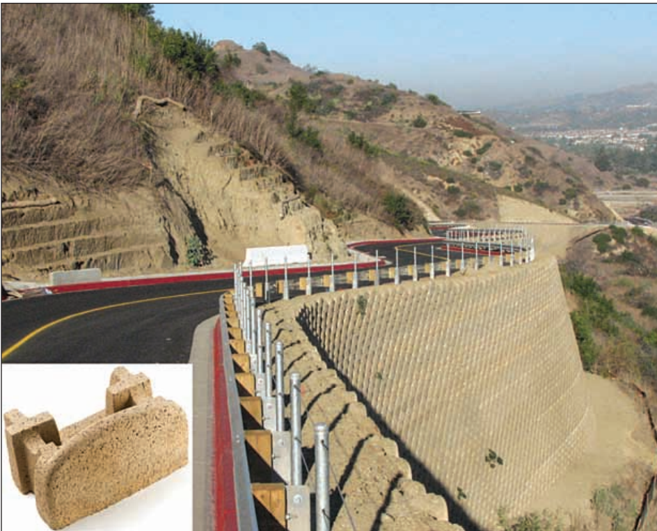
Close-up of Soil Retention's Verdura® wall for the north access road to the Robert B. Diemer Water Treatment Plant in Yorba Linda, CA.
