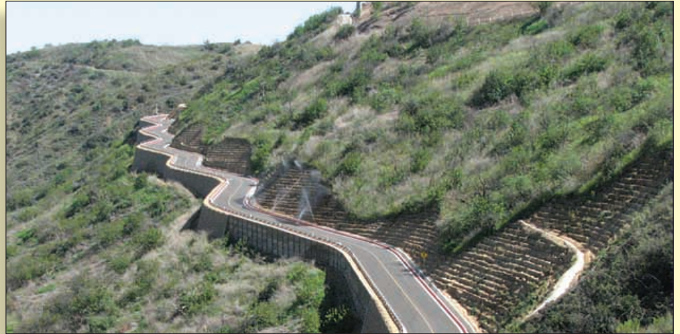
Soil Retention offers concrete systems that can be combined with vegetation to soften the overall look: See page 16
