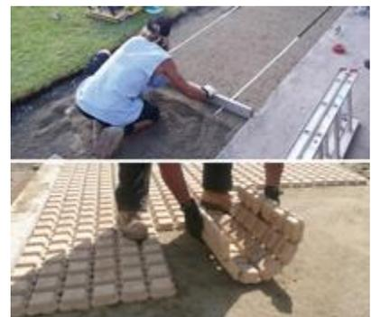
The grid inside the Drivable Grass® mats can be cut with a utility knife or chisel to fit site conditions. At terminating edges or curved installations, the mats should be fit with a masonry blade on a rotary saw.
